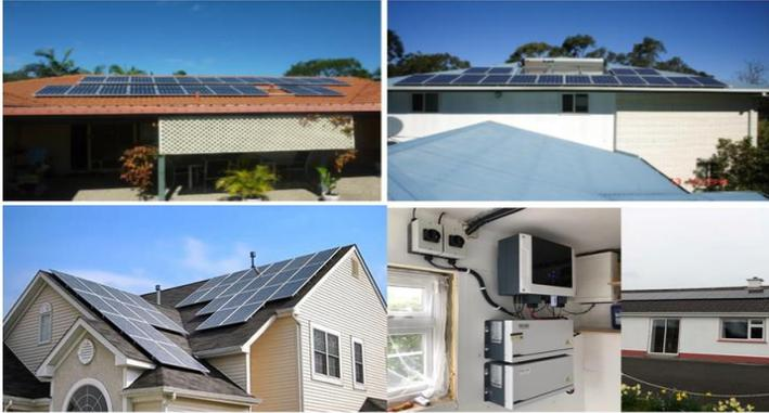
**Figure 3 Photovoltaic solar energy installations connected alongside with the batteries and inverter for residential applications (Ohwofasa, 2018)**
